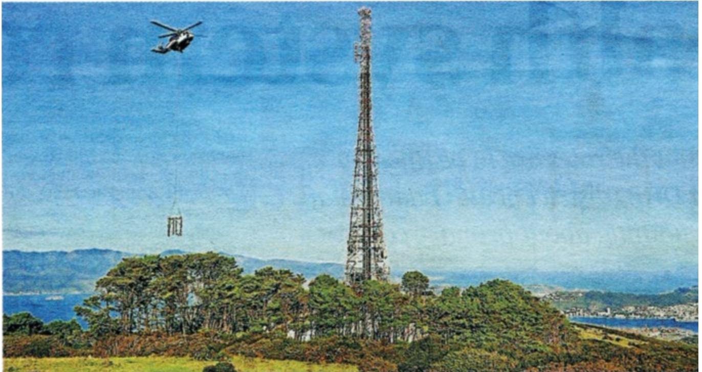
After 60 years, the top part of the aerial on Mt Kaukau in Wellington is removed by helicopter. It is the most visible high point in the Wellington landscape. PHOTO: KORDIA
